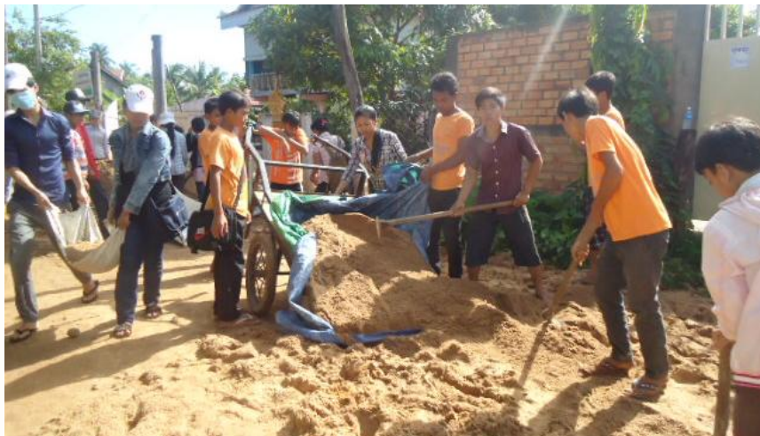
(KBFC's Youth Club constructing a village road)
