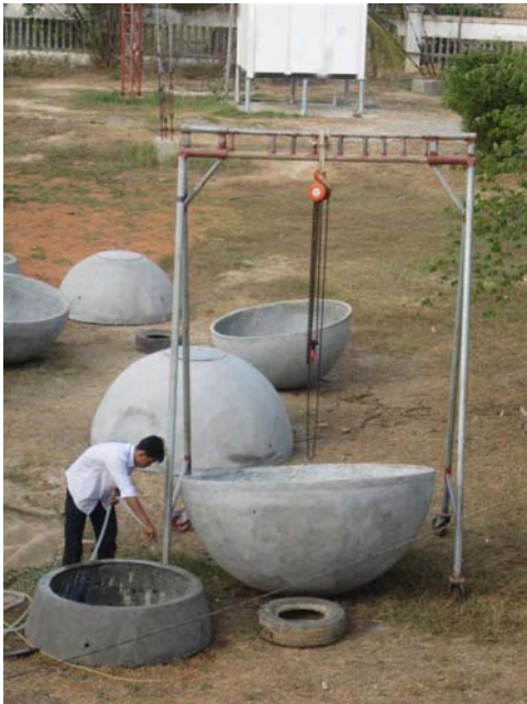
Building a RRH Container
